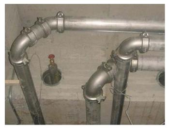
Shurjoint Model SS-8 2.5" austenitic grade CF8M (316) stainless steel couplings were selected and specified in the glycol pipeline because of their cost, quality, durability and ease of maintenance. In addition, Shurjoint #SS-8 Couplings are UL listed and FM approved. location
